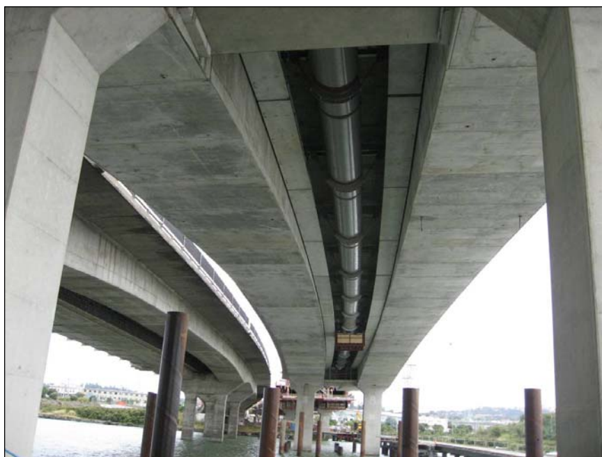
The Manukau Harbour Crossing section of the Hunua No. 4 Water Supply Scheme project.
